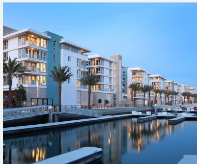
NEPTUNE AT MARINA DEL RAY Los Angeles, CA 97% Occupancy
